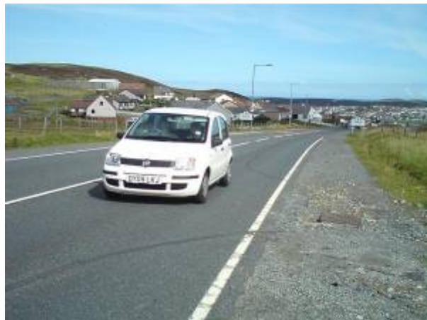
Completed application into a service chamber
